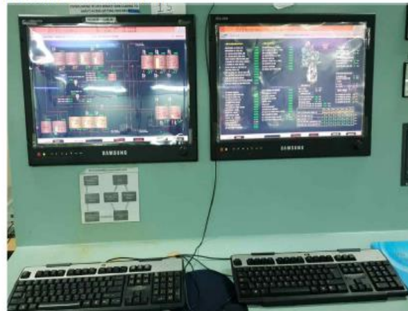
NK -BULE BALLAST SYSTEM MAIN CONTROL PANEL (Position : Steering Gear Room) AMS MAIN MONITOR (Position : Engin Control Room) # NK BWTS Valve Signal
